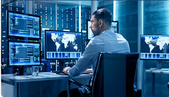
NOC (Network Operation Center)
